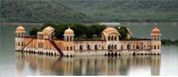
JAL MAHAL PROJECT, JAIPUR
